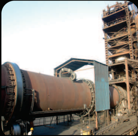
Coal Based DRI Plant
