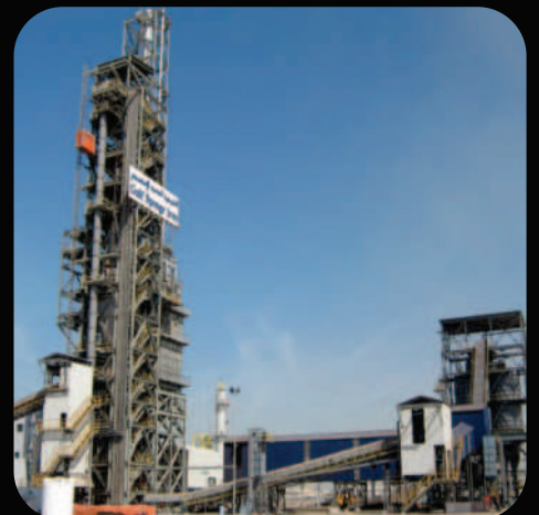
Gas based DRI Plant
