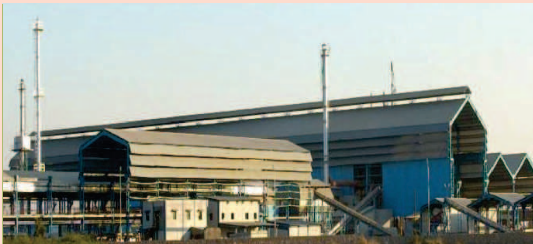
Plant at Samakhiali, Kutch
