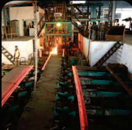
Continuous Casting Machine
